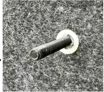
Install nylon washers onto studs
